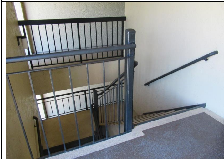
6. Handrails in Stairwell
