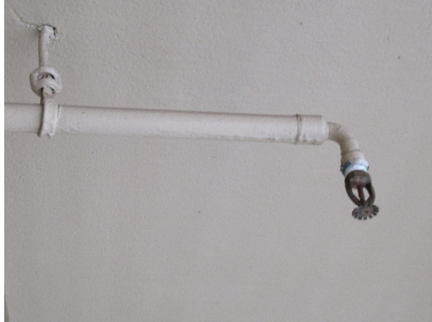
Typical fire suppression sprinkler head
