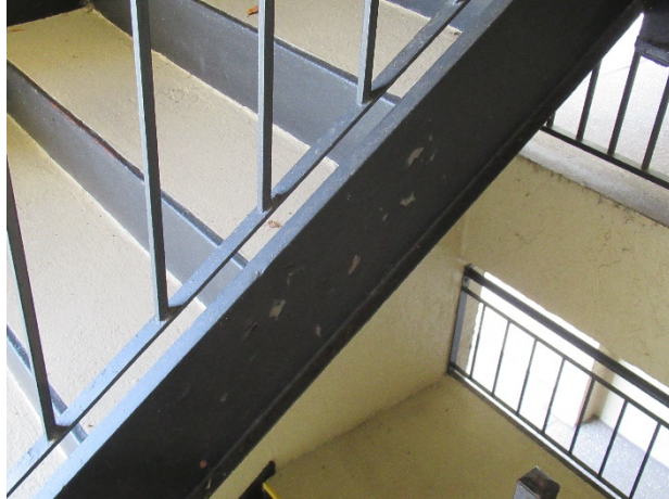
Peeling paint at staircase
