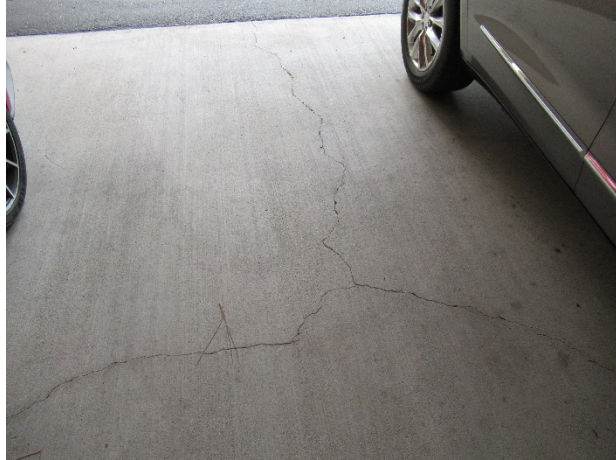
Concrete crack at garage
