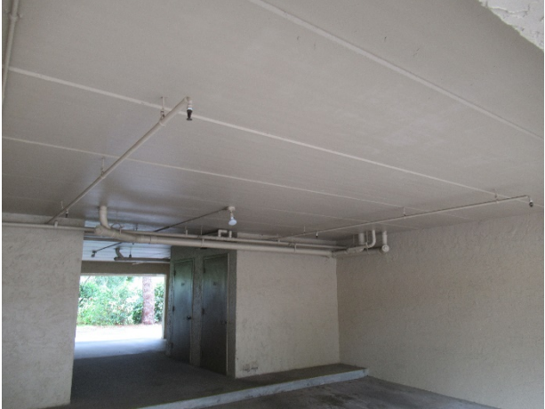
Typical fire suppression system at garage
