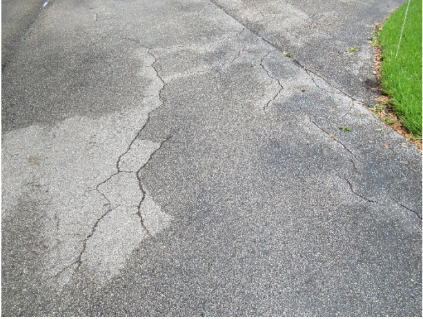
Asphalt pavement cracks
