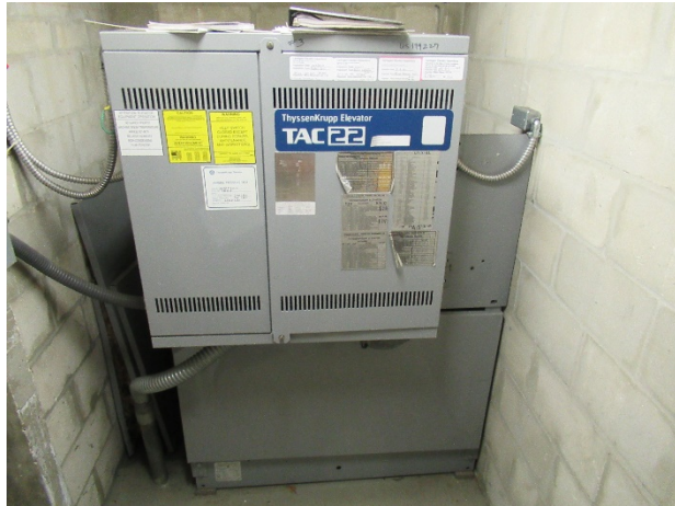
Pump housing and controller
