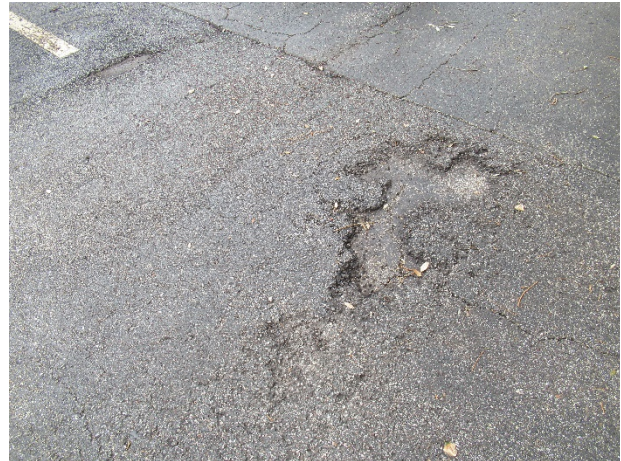
Cracks and raveling at pavement
