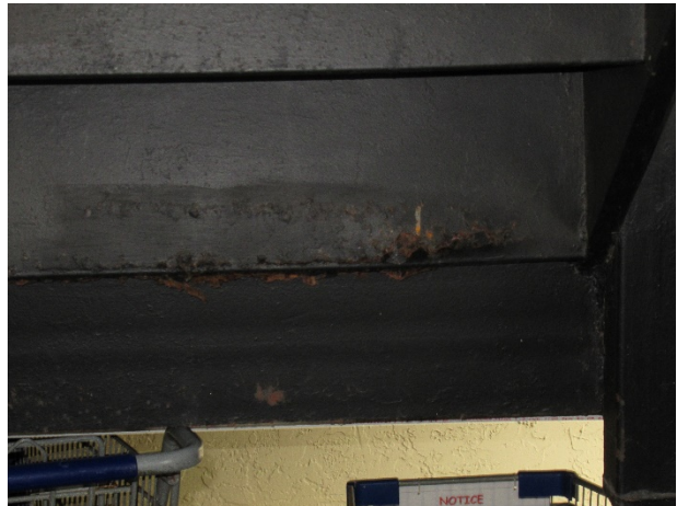
Heavy rust at staircase
