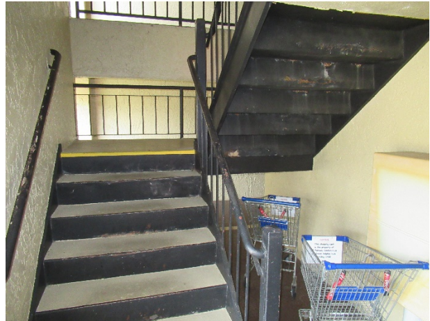
Staircase with widespread rust
