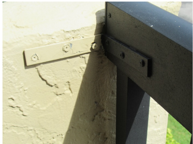
Previous repair at breezeway railing
