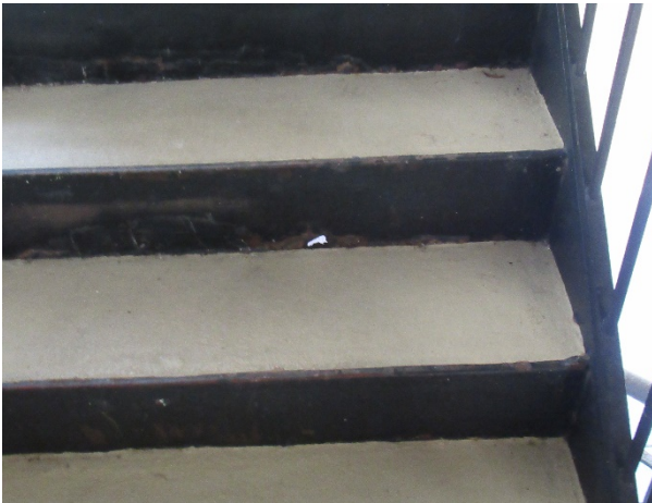
Staircase with rusted through hole
