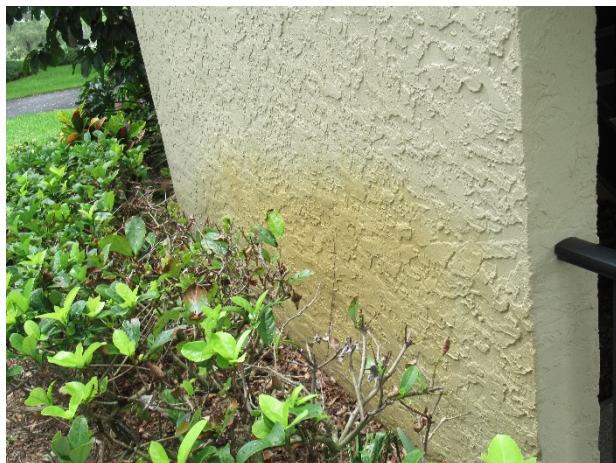
Isolated stain at stucco wall
