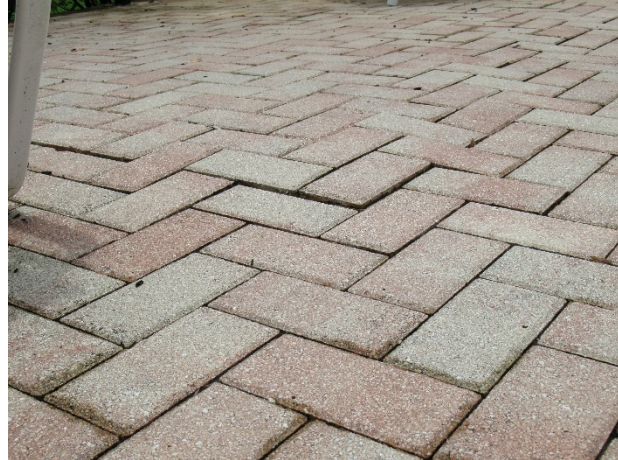
Minor settlement at pool deck pavers
