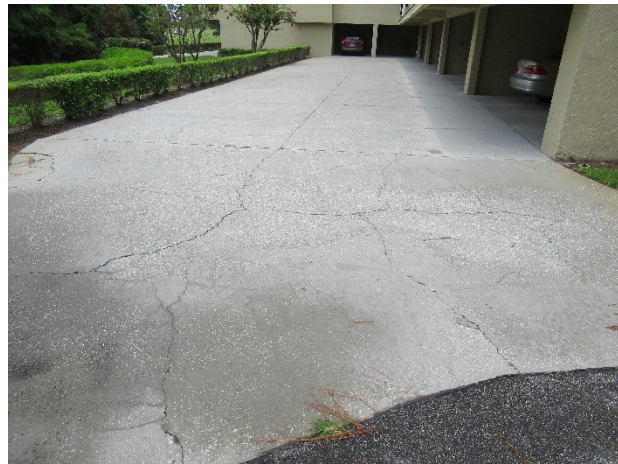
Concrete driveway with cracks
