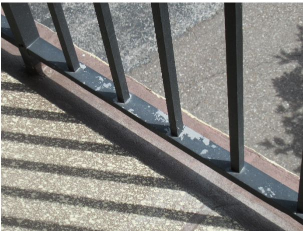
Breezeway railing finish deterioration
