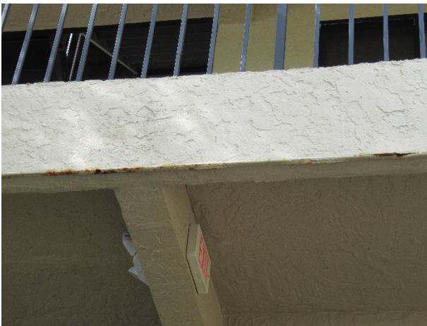
Signs of water intrusion with rust
