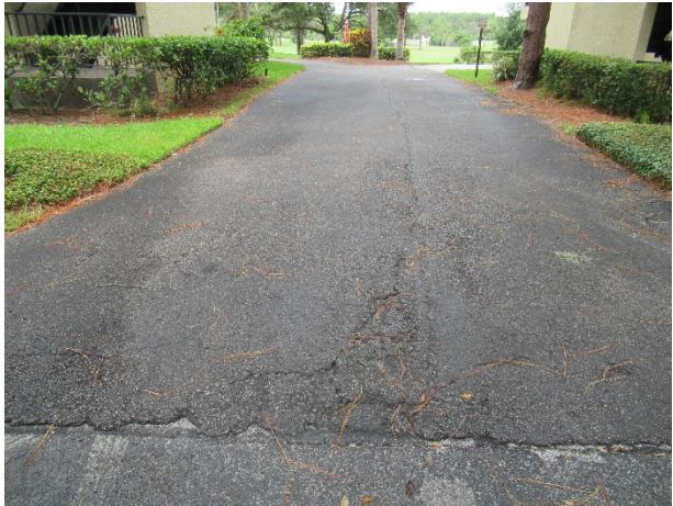
Cracks and raveling at pavement
