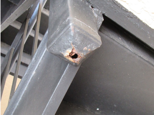
Rusted staircase component
