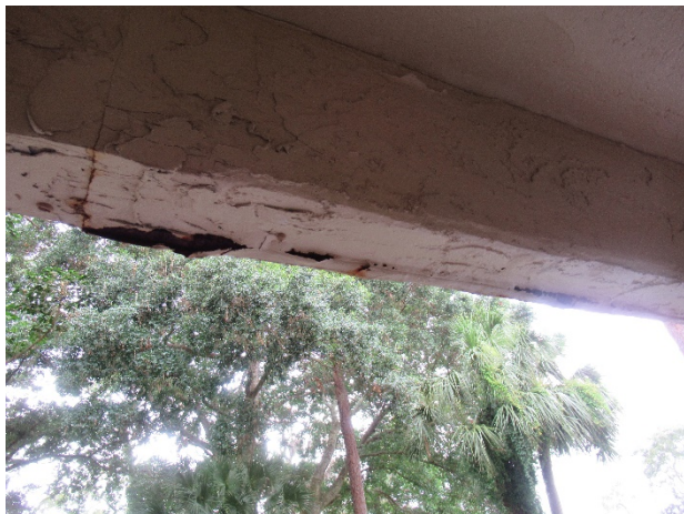
Signs of water intrusion with rust
