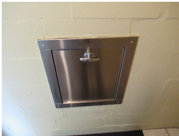
Typical trash chute door
