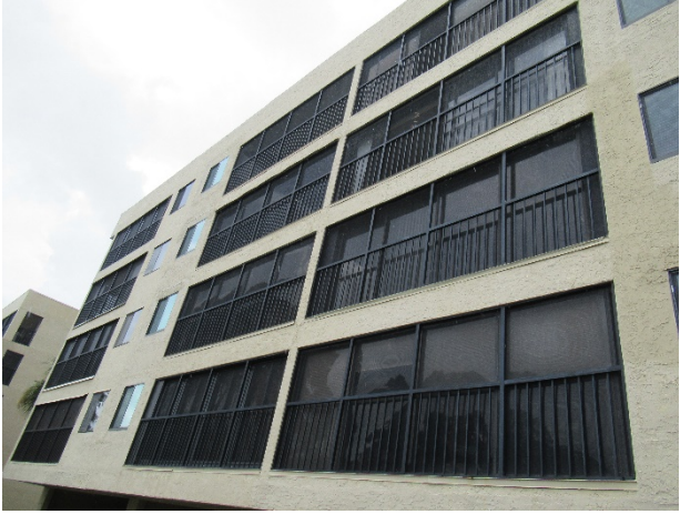
Typical balcony railings with screen enclosures
