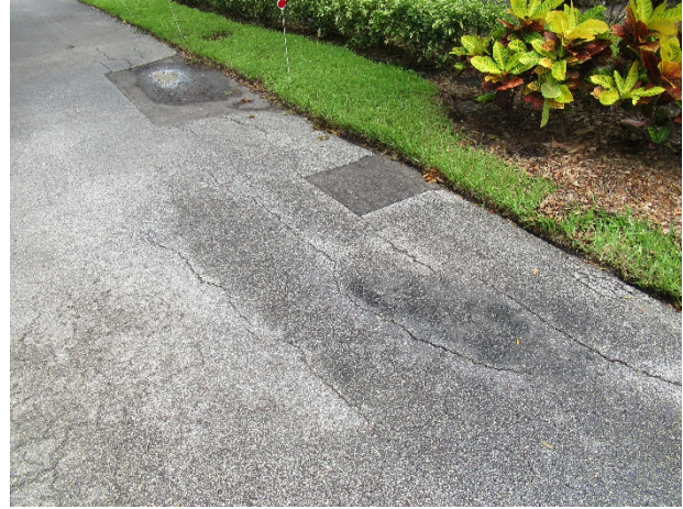
Longitudinal cracks, patches and settlement
