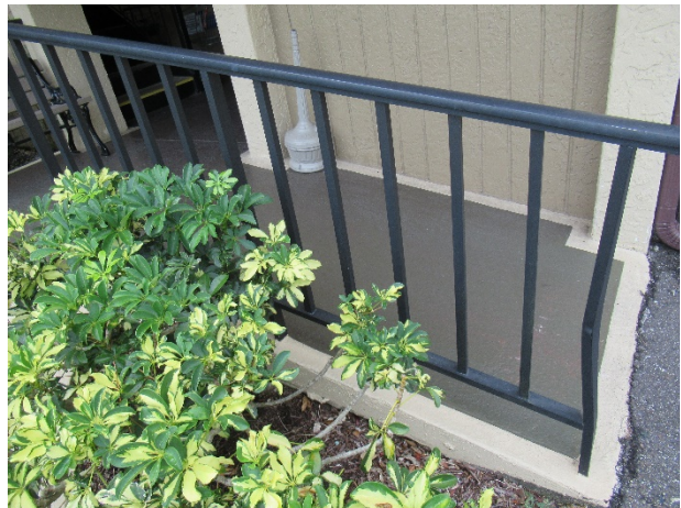
Breezeway railing with bent picket
