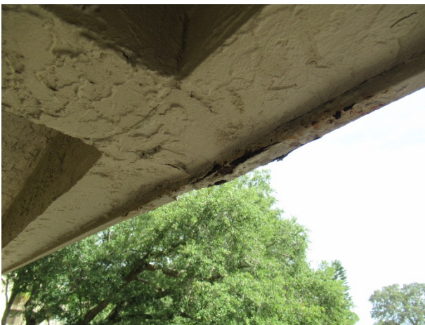
Signs of water intrusion with rust
