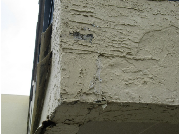
Isolated wall coating deterioration
