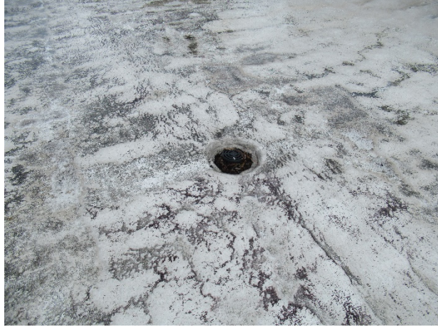
Typical drain at foam roof
