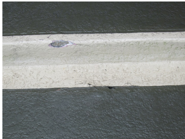
Coating damage at breezeway
