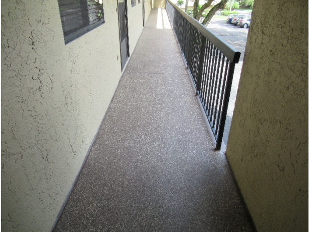
Typical breezeway and waterproof coating
