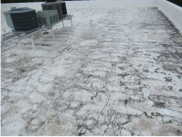
Typical foam roof
