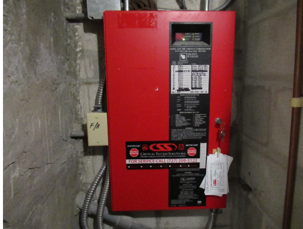
Life safety system control panel
