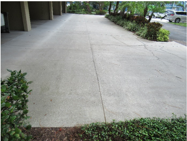
Concrete driveway with cracks
