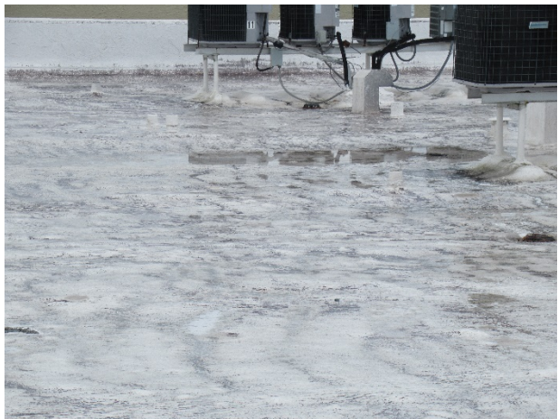
Standing water at foam roof
