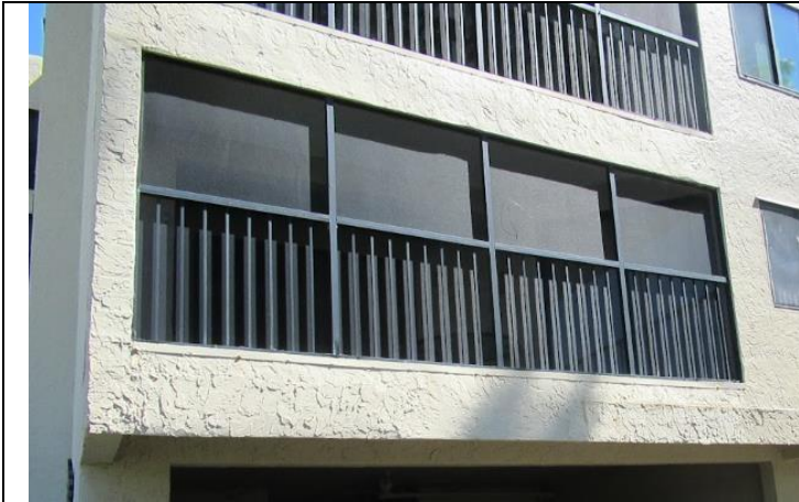
8. Unit Balcony Guard Rail (typical)
