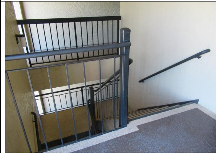
6. Handrails in Stairwell
